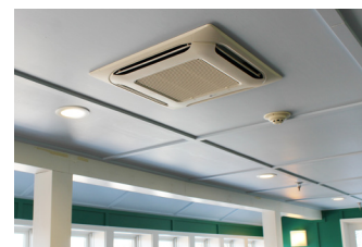
The Mass Audubon Joppa Flats facility utilizes ceiling vents throughout the building to evenly distribute heating or cooling.
